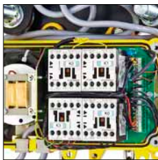
Increased operating safety through 42 V control voltage
